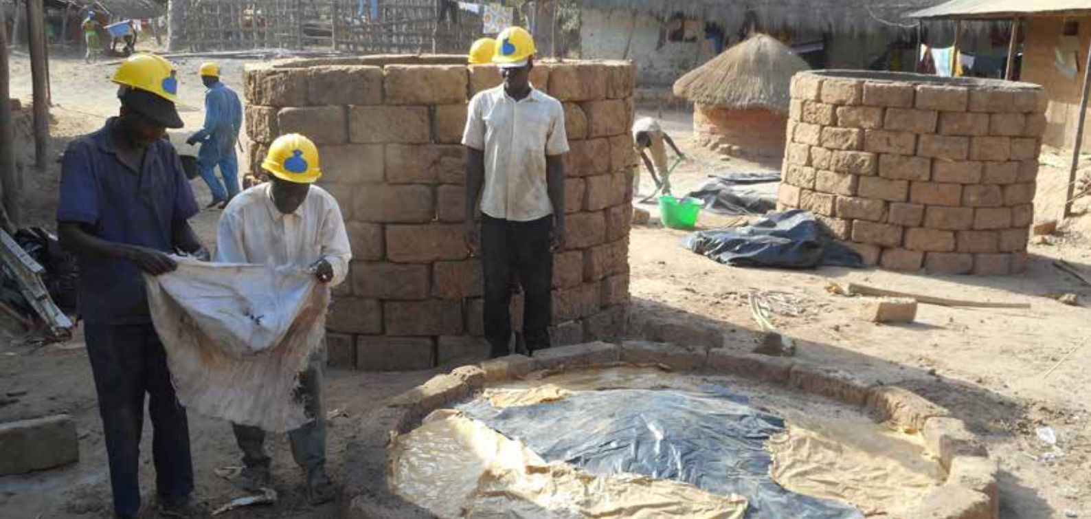
Above: watertanks under construction. Under: same tanks ready for use.
